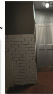
Industrial clean & redecorate toilets
