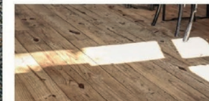
Clean & polish timber floor
