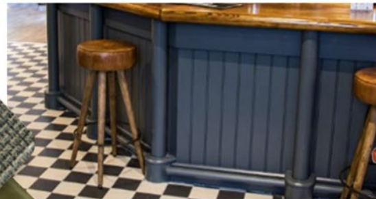
Add new pilasters to bar counter to break up front and paint inset t&g.
