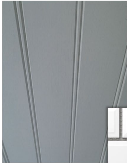
Cubicles And Vanity Unit Front
