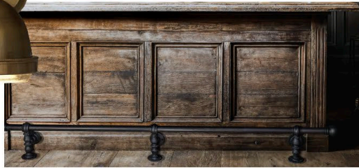
Distressed Finish To Existing Bar Front
