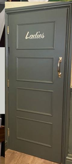
applied mouldings to toilet doors
